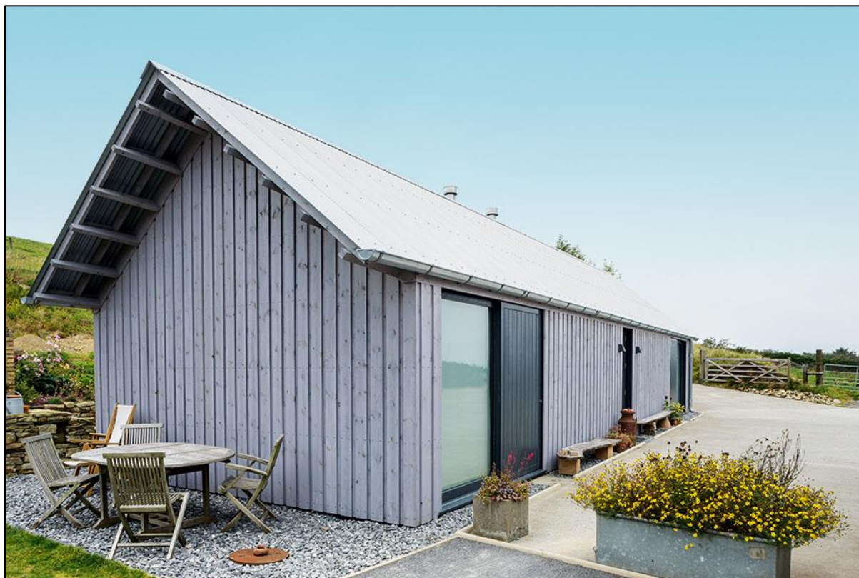
An example of a small single storey, affordable and secure barn style building 78
